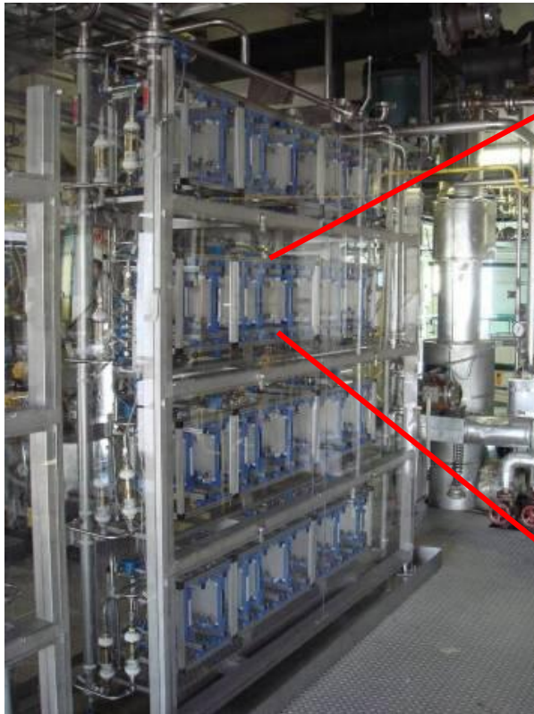
2 towers with 4 lines each 96 micro reactors in total
